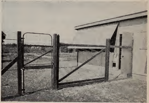
Fig. 65. An 8-foot removable fence panel provides driveway in front of poultry house.
